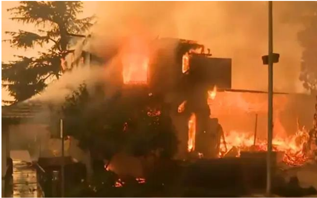
Photograph of the Eaton Fire destroying the Altadena Senior Center 7
