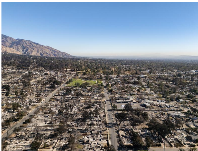
27 Aerial footage depicting widespread devastation from the Eaton Fire in Altadena
