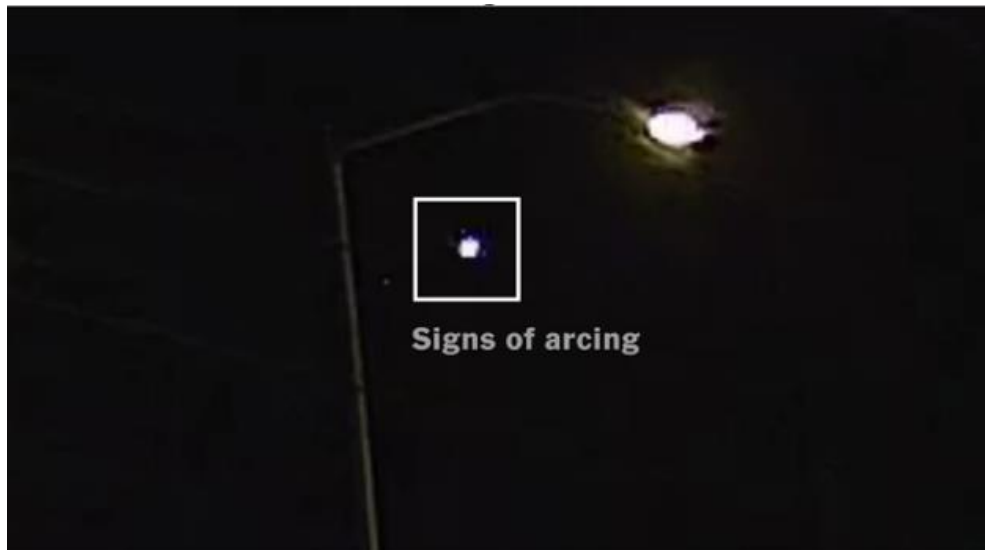
Still photographs of video footage capturing electrical arcing events on EDISON’s transmission towers moments before the Eaton Fire ignited 9
