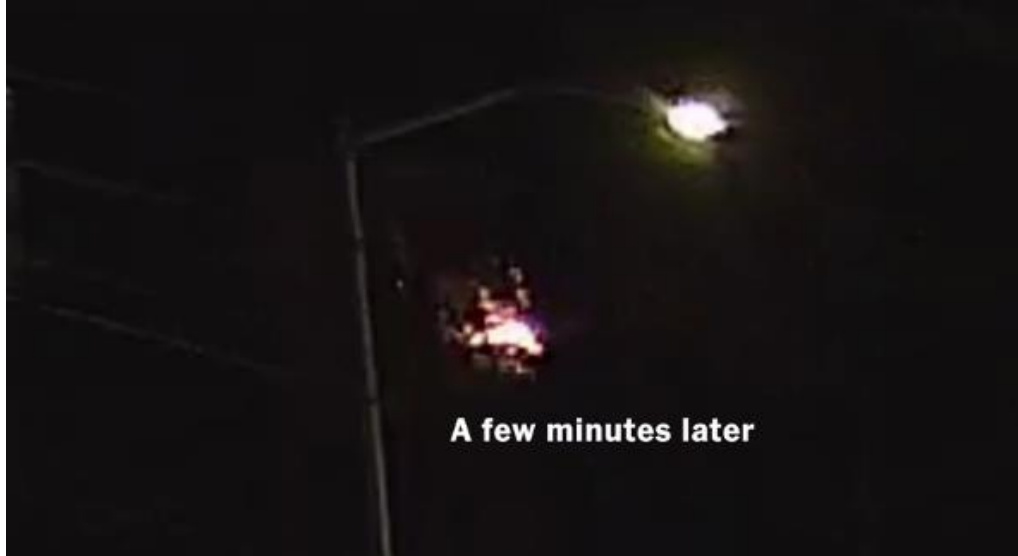
10 Still photographs of video footage capturing electrical arcing events and resulting flames under EDISON's transmission towers 10
